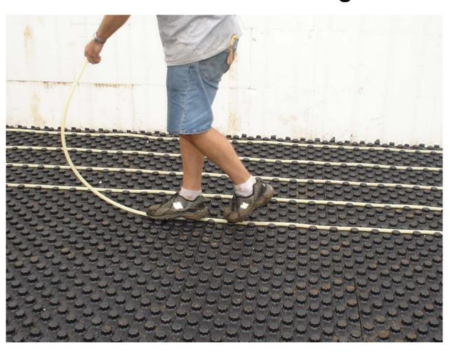
The RAZ Panel<sup>™</sup> modular board system from EZ Floor, LLC is an easily installed vapor barrier, insulation board and PEX tube holder all in one. This product allows for simple installation of hydronic radiant floor heating systems that today consist of primarily garages, basements and slab-ongrade installations where concrete is used.
