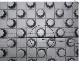
NOTE: The panels are divided into 2" squares. Each square either contains a knob or a flat and they alternate every other square. When placing the first panel of a new row you must check to verify that from row to row, this alternating sequence of knobflat-knob-flat is not interrupted.
