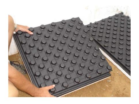
The reason for the preceding step is twofold. First, we want to make sure that we stager the joints where panels come together to avoid common seams.
