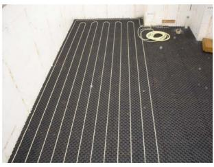
Other than ensuring the PEX is securely in the panel when making a corner, installation is as simple as walking the tube into place.
