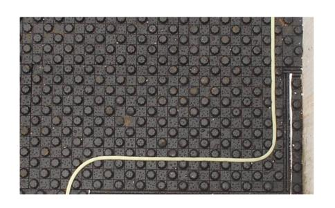
The only tip about making the PEX installation easier is that when making a turn, ensure the PEX is fully seated in the knobs before beginning or continuing a run.
