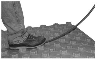
• The only tip about making the PEX installation easier is that when making a turn, ensure the PEX is fully seated in the knobs before
