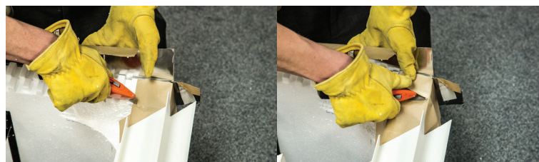
The stainless steel barrier wraps around the interior and exterior flange. Form a tight seal around the flange radius.
