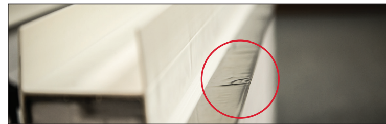
The stainless steel barrier wraps around the interior and exterior flange. Form a tight seal around the flange radius.
