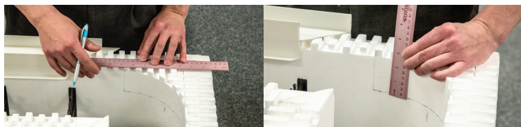
Figure 2. Corner form modified to remove foam radius in corner for BuildShield installation. Note radius is only removed to a depth of 3". Corner form modified to remove interlock fingers and foam radius removed in corner for BuildShield installation. Note this form is placed with the modifications toward the BuildShield Extrusion Track.
