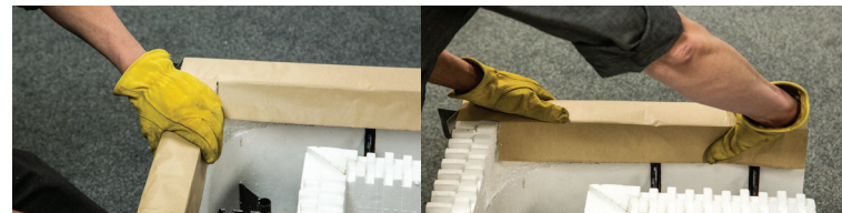
Figure 2. Corner form modified to remove foam radius in corner for BuildShield installation. Note radius is only removed to a depth of 3". Corner form modified to remove interlock fingers and foam radius removed in corner for BuildShield installation. Note this form is placed with the modifications toward the BuildShield Extrusion Track.
