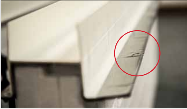
The stainless steel barrier wraps around the interior and exterior flange. Form a tight seal around the flange radius.
