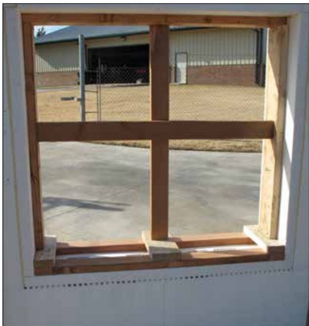
Figure 2.5 Fully cross braced 4040 rough opening.
