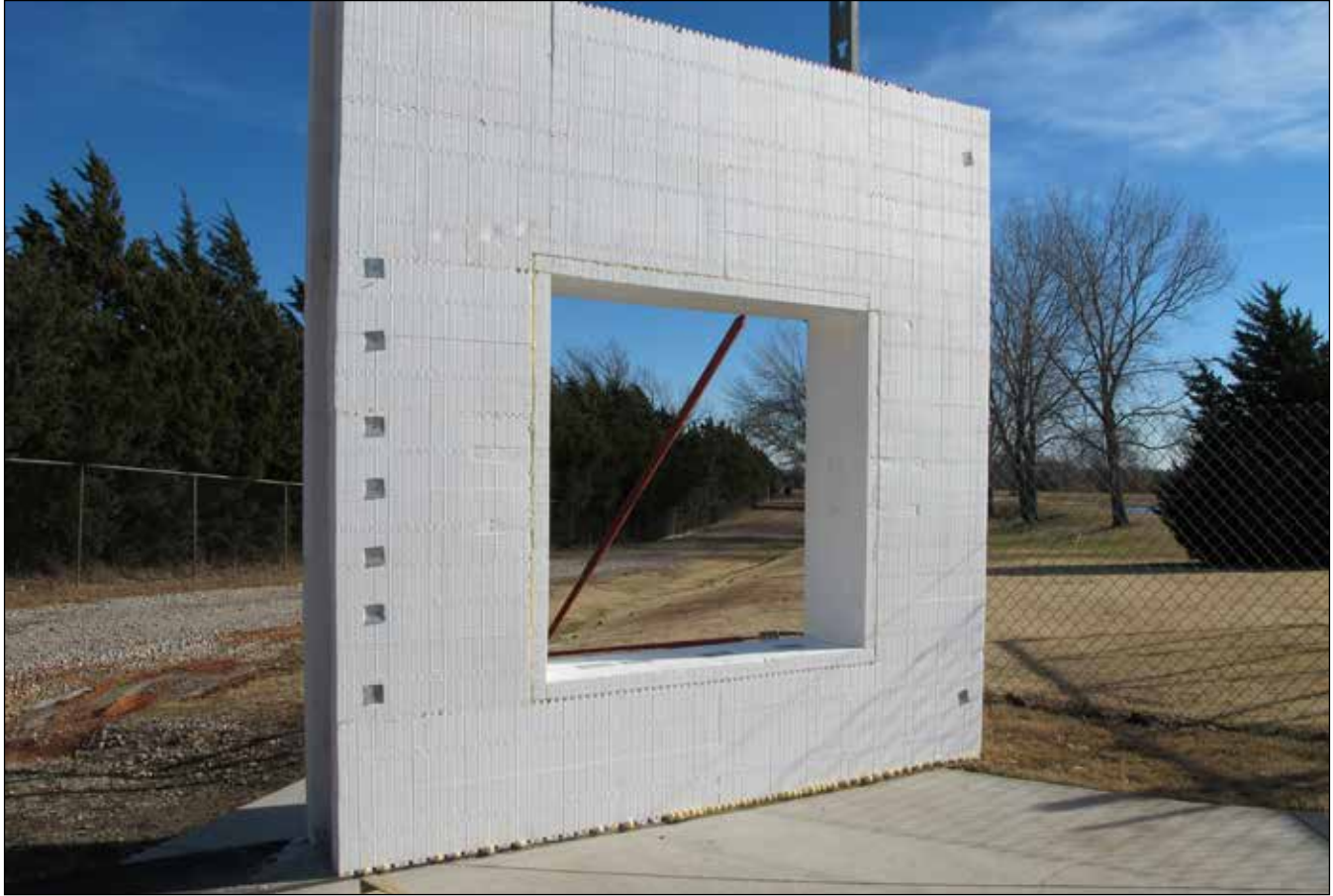
Figure 2.1 BuildBuck poured and bracing remove after concrete fully cured.
