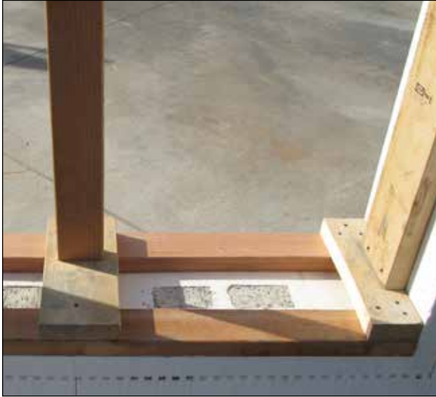
Figure 2.3 Concrete window inspection ports fully filled.
