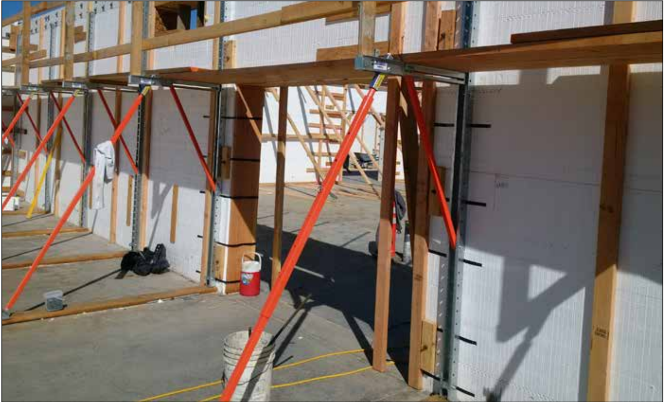
BuildBrace Build1 ICF Bracing.
