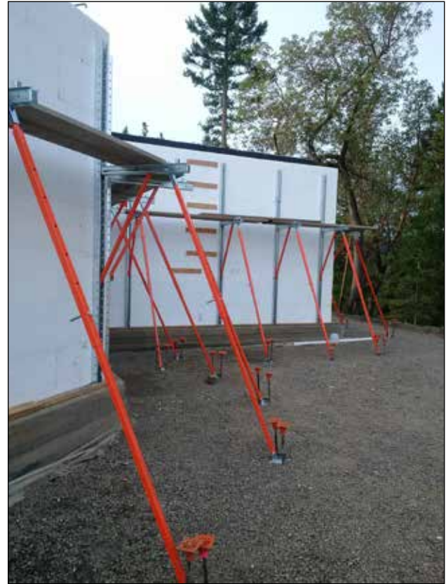
BuildBrace Build1 erected and staked.
