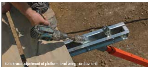
BuildBrace adjustment at platform level using cordless drill.
