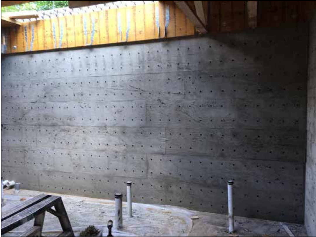
Figure 1.6 Poured BuildBlock HardWall wall with formboard removed.
