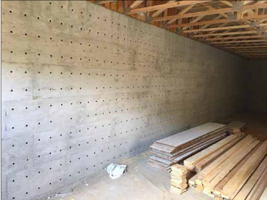
Figure 1.7 Poured BuildBlock HardWall wall with formboard removed and ready for finishes.
