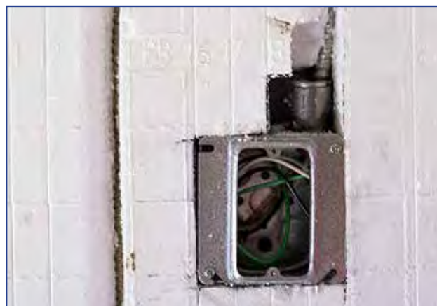
Figure 11.1.4 Electrical box with small wire chase cut in foam.
