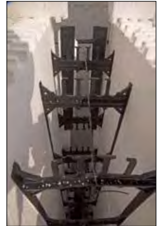
Figure 5.5.7 Intersecting wall opening cavity and wire tied to secure forms.
