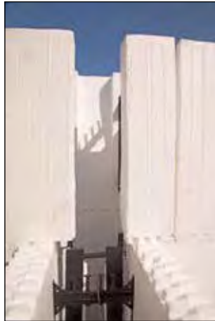
Figure 5.5.5 Intersecting wall opening alternating form placement.
