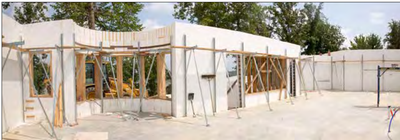
BuildBlock ICF Interior walls braced and ready for pouring.
