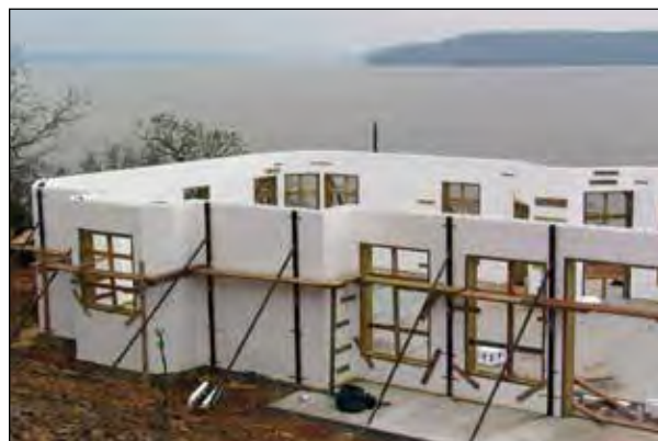
Figure 9.6.1 Minimal Outer Bracing
