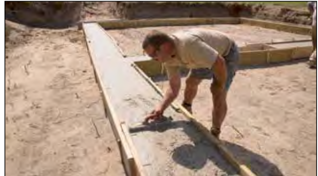
Figure 4.1.7 Level footings to the correct height and ensure a smooth finish.
