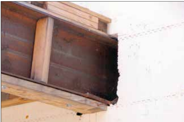
Figure 5.11.1 Steel beam placed in ICF beam pocket.
