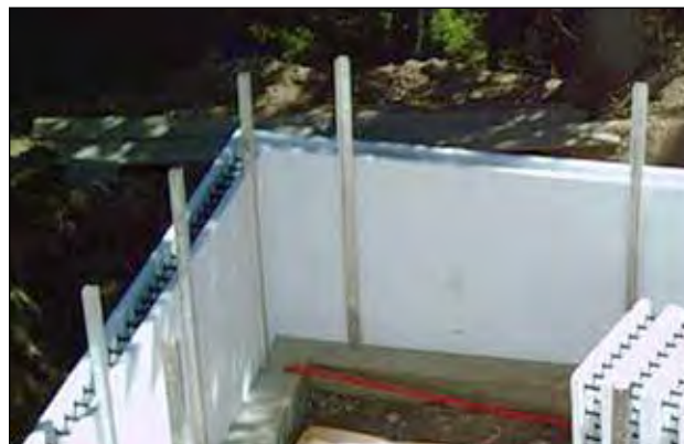
Figure 9.6.3 Minimal Inner Bracing
