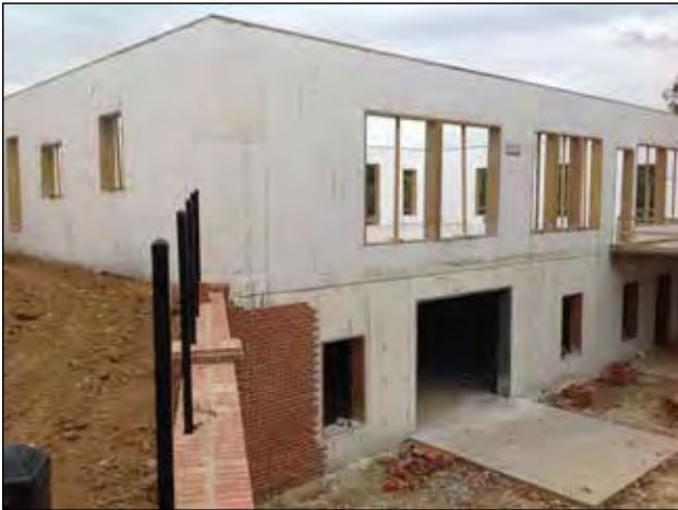
Figure 3.5.1 Lintels above multiple door and window openings in a residential home.
