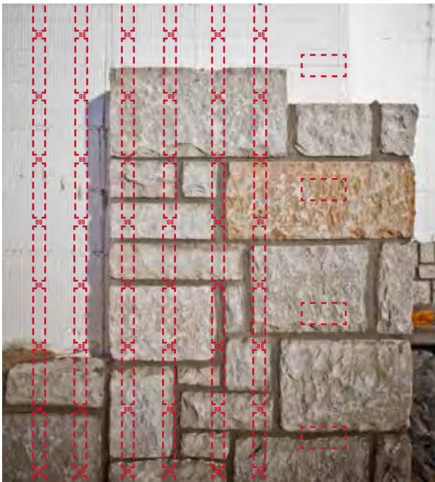
Figure 11.1.1 BuildBlock ICF wall showing standard and heavy-duty attachment points with webs correctly aligned.
