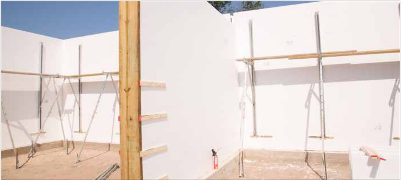
Figure 6.2.1 ICF walkout basement and garage braced and poured.
