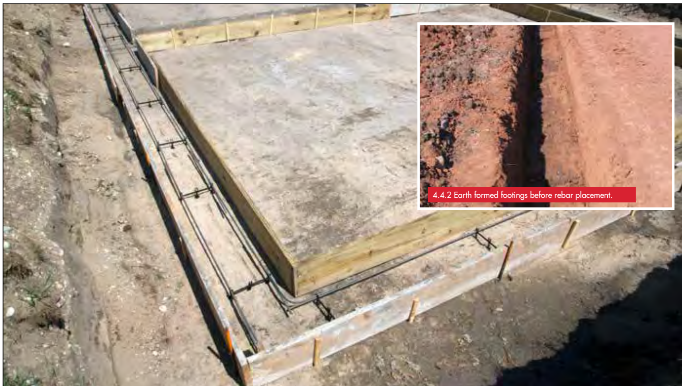
Figure 4.4.1 Footings formed with horizontal rebar in place.
