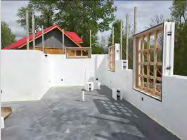
Figure 8.4.1 ICF Foam Bucking placed in the wall and cross-braced appropriately.
