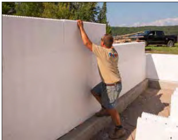
Figure 4.5.1 Stacking ICF walls using spot glued dry set method.
