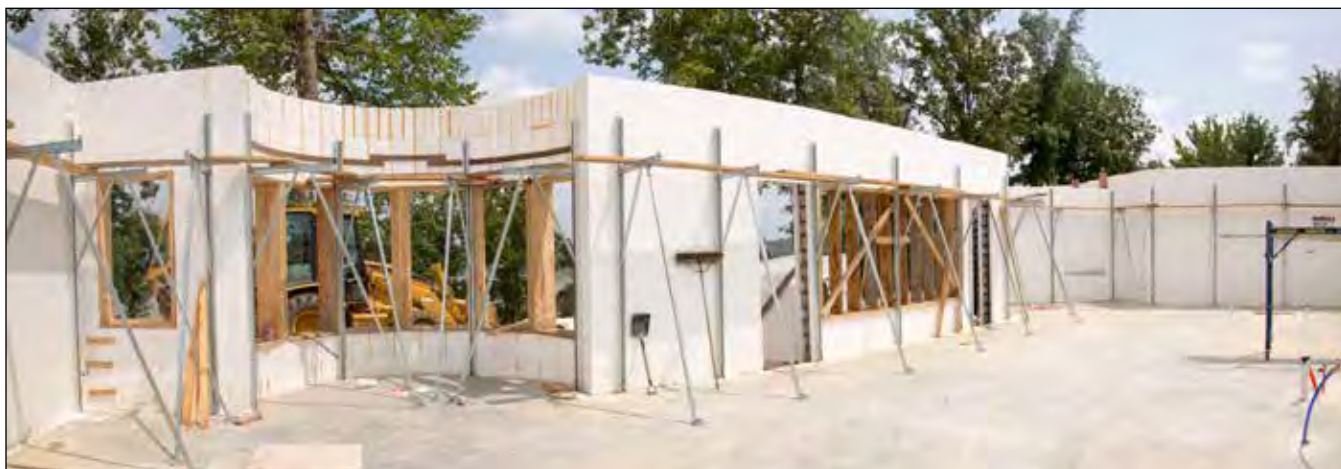
Figure 8.1.1 ICF walls braced and windows bucked before a pour.
