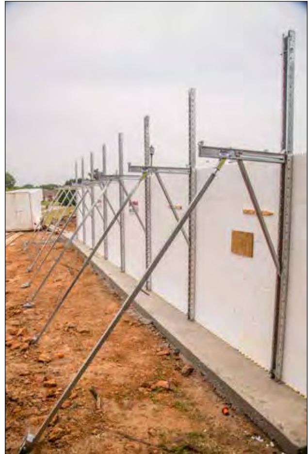
Figure 4.5.3 BuildBlock Build1 ICF bracing and alignment system set up with proper spacing.
