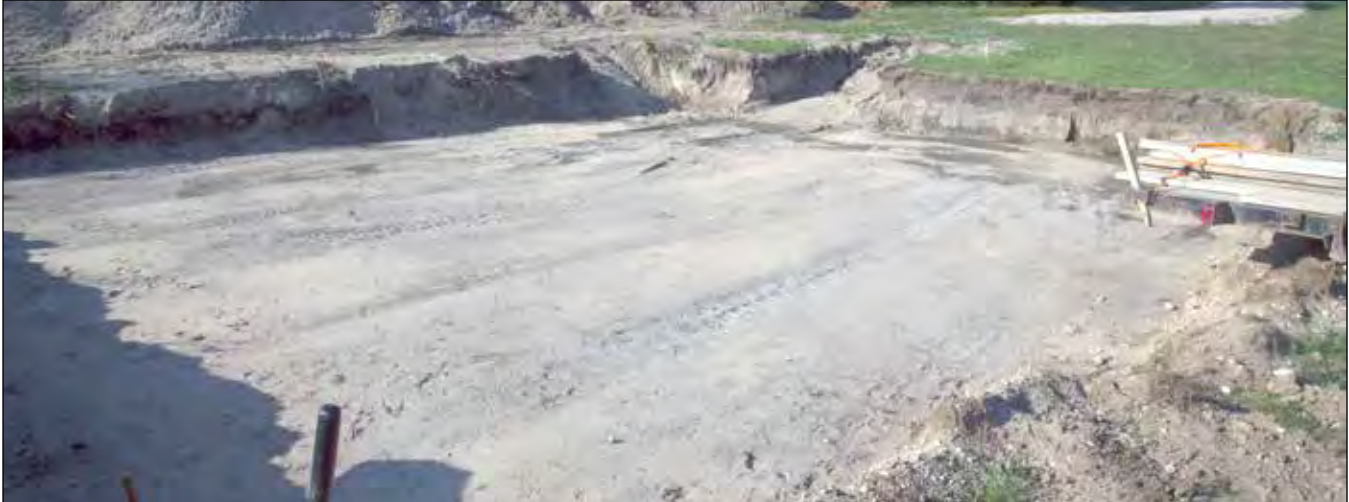
Figure 4.2.1 Typical site excavation staked for square
