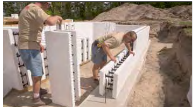
Figure 4.1.9 A smooth level finish will make stacking and leveling the ICF wall easier.
