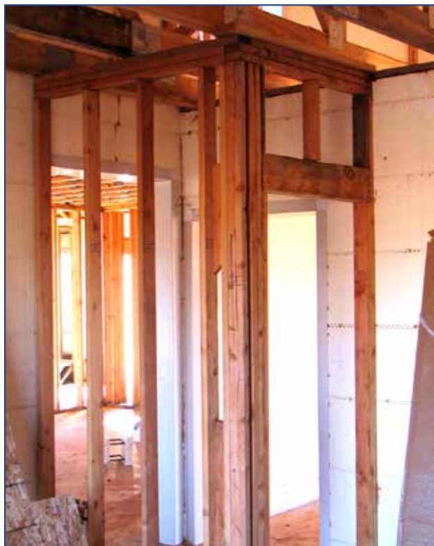
Figure 11.1.3 Internal wood framing is attached to BuildBlock ICF walls with screws. Tapcons can also be used if needed.
