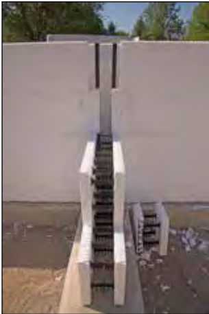
Figure 5.5.4 Intersecting wall opening types.
