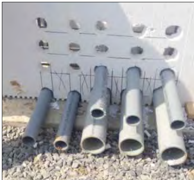
Figure 7.1.1 Complex service penetrations before additional strapping.
