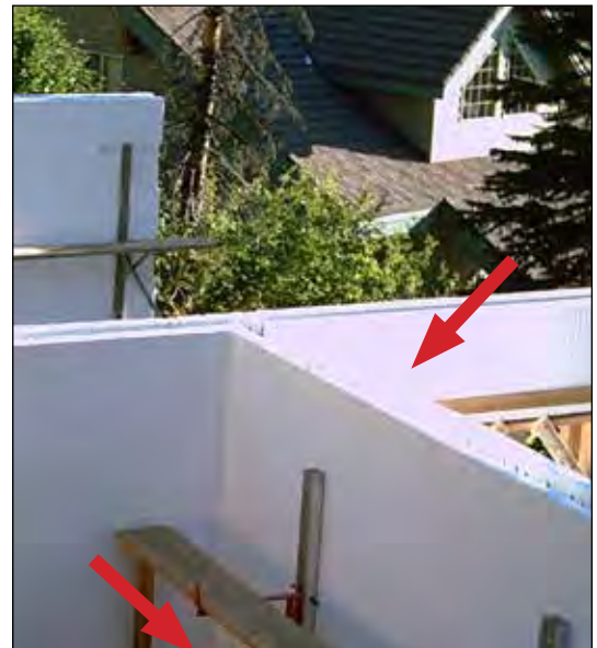
Figure 5.5.9 Intersecting wall opening types.
