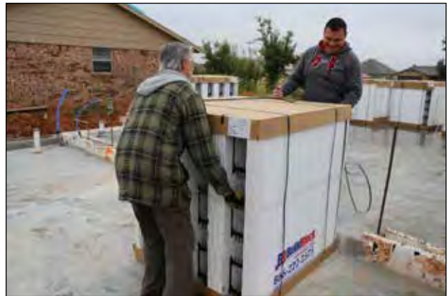
Figure 1.7.3 BuildBlock forms are easily moved around a job site by 1 or two people Drag do not roll to prevent damaging interlock or edges.
