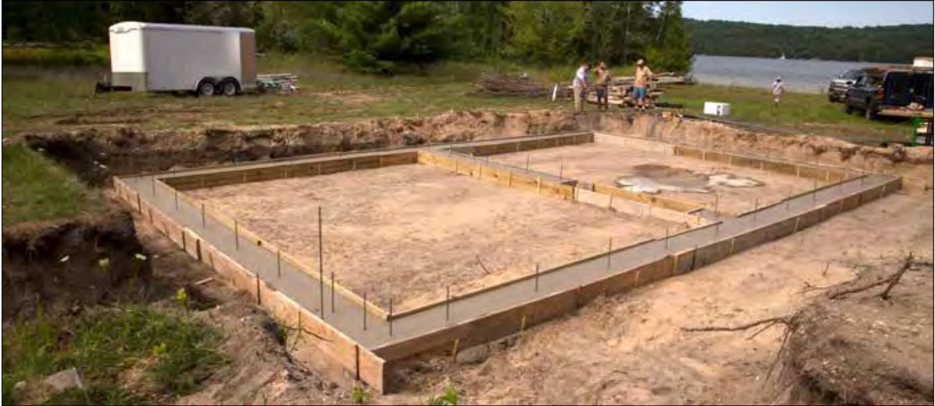
Figure 4.1.1 Typical footing layout with vertical rebar dowels placed.
