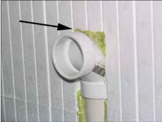
Figure 11.1.7 2" PVC pipe chased into an ICF wall.
