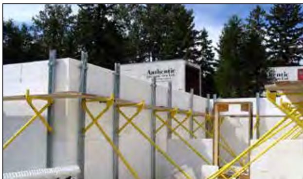
Figure 9.6.4 More Secure Inner Bracing w/ Walk Board
