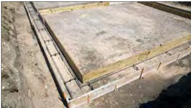
Figure 4.1.5 Formed footings with horizontal rebar placed in per local codes.
