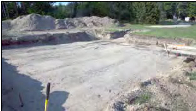
Figure 4.1.4 Excavated Footprint for footings.
