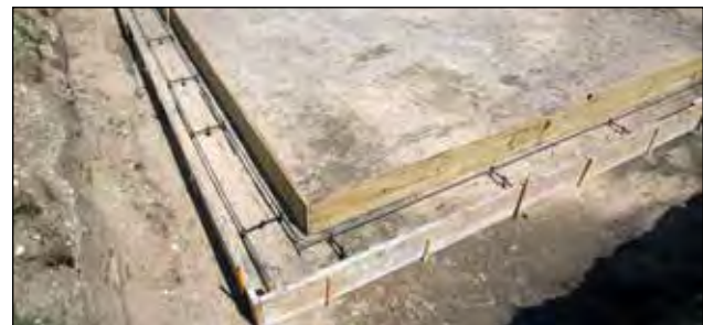
Figure 4.2.2 Formed and reinforced footings ready for pouring.
