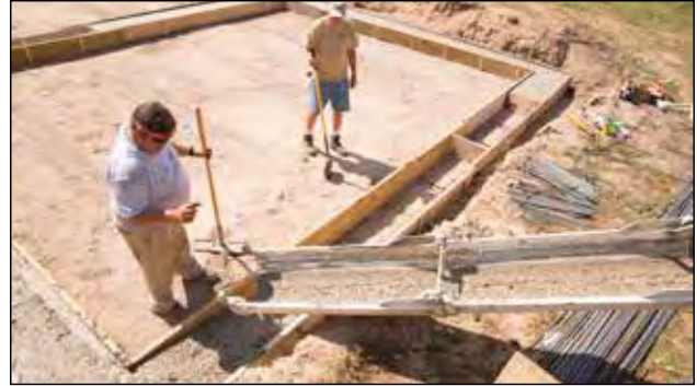
Figure 4.1.6 Pour footings and ensure good consolidation and a smooth finish.
