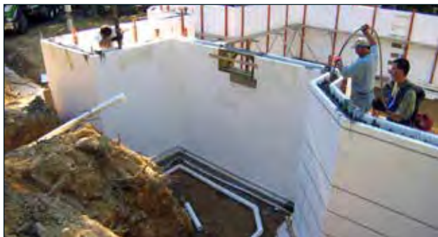
Figure 6.1.2 Standard french drain using slotted PVC pipe:
