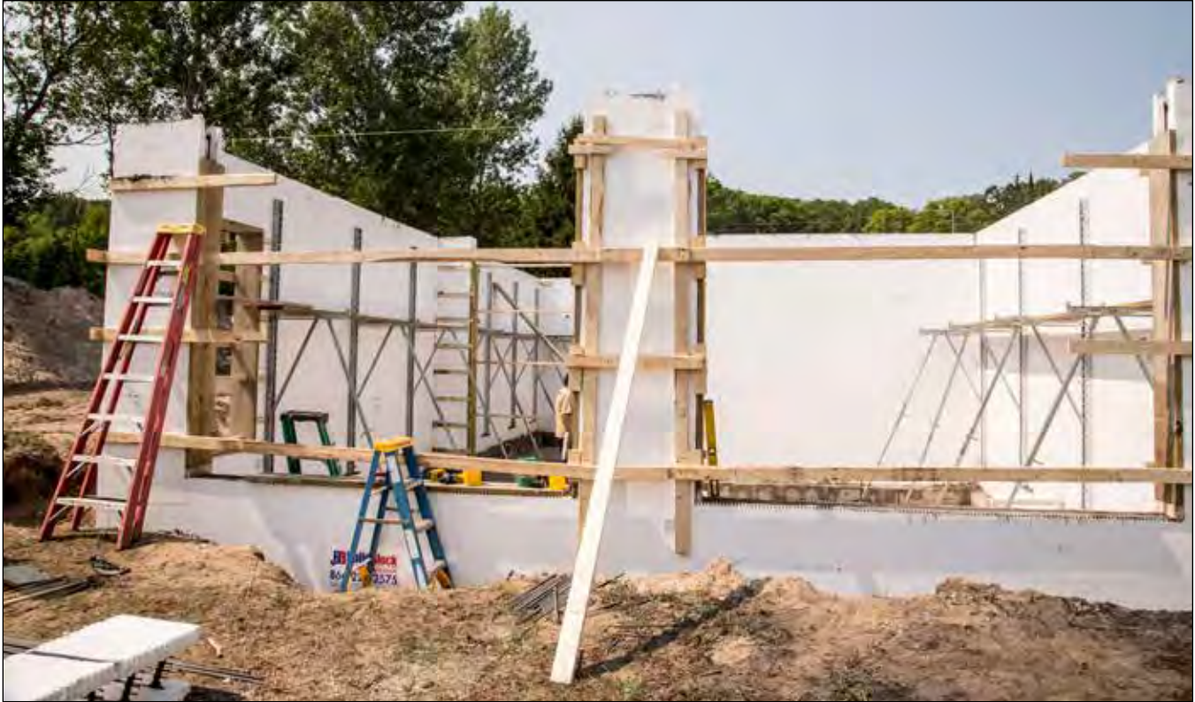
Figure 4.5.2 Walls stacked, braced, and prepped before pouring walls.
