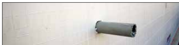
Figure 7.1.4 Secure any space around the pipe sleeve with foam adhesive before the pour.
