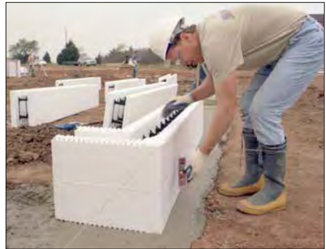
Figure 4.3.3 Placing corner forms during a wet set. (See CAD Details 6, 7 and 8.)
