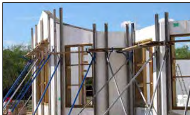
Figure 9.6.2 More Secure Outer Bracing
